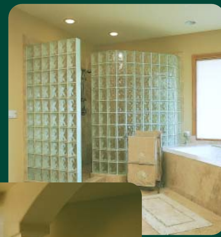
Abbott Custom Homes Spec home Seattle Glass Block Design Decora® Pattern Arque® radius blocks used to make 45° angles. Style cap finished ends.
